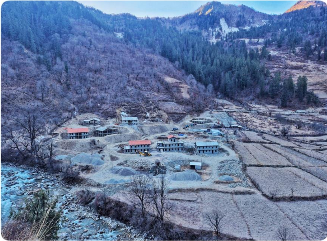
CONSTRUCTION OF THE CAMP FACILITY AT HEADWORKS SITE
