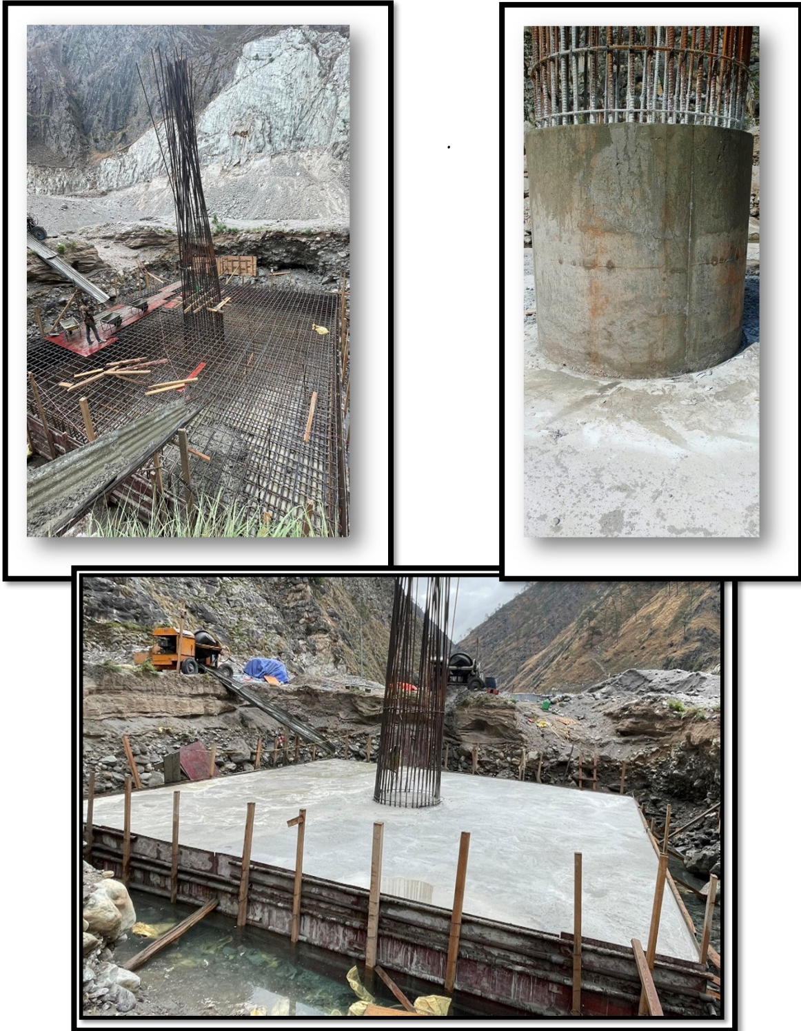
Figure 31: Construction preparation of RCC Bridge Pier
