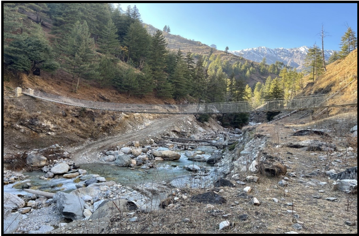
Figure 44: Blasting area of the Access Road to the Project Site
