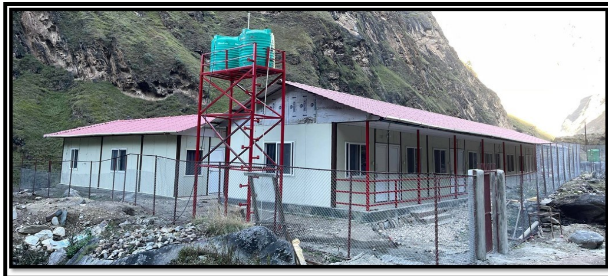
Figure 11: Completed Prefab Office cum Residential Building
