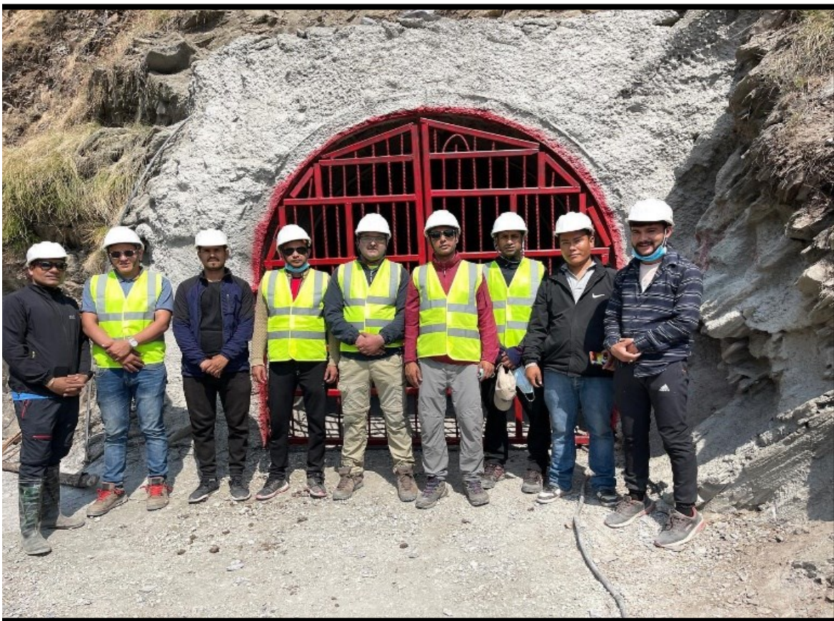
Figure 8: Test Tunnel Completed
