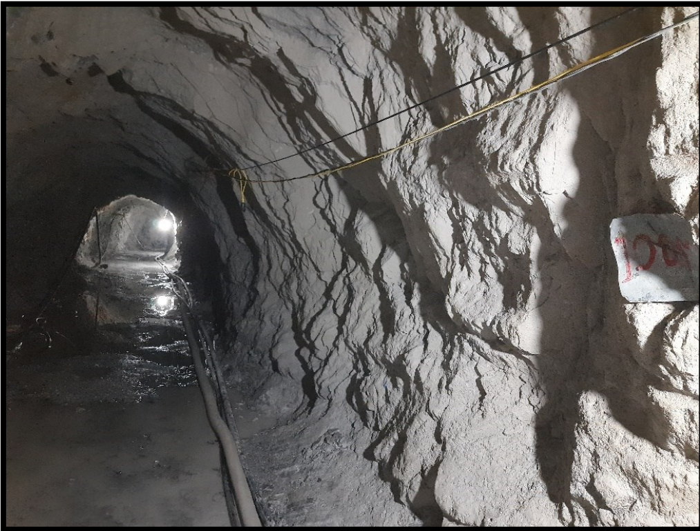
Figure 10: Test Tunnel Photos
