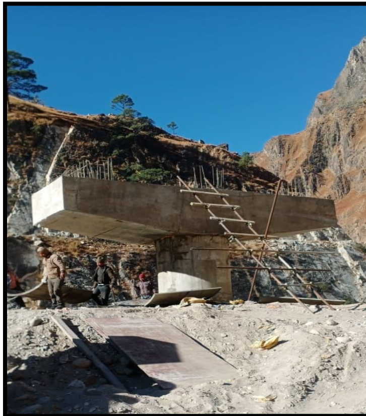
Figure 32: Construction preparation of RCC Bridge Pier
