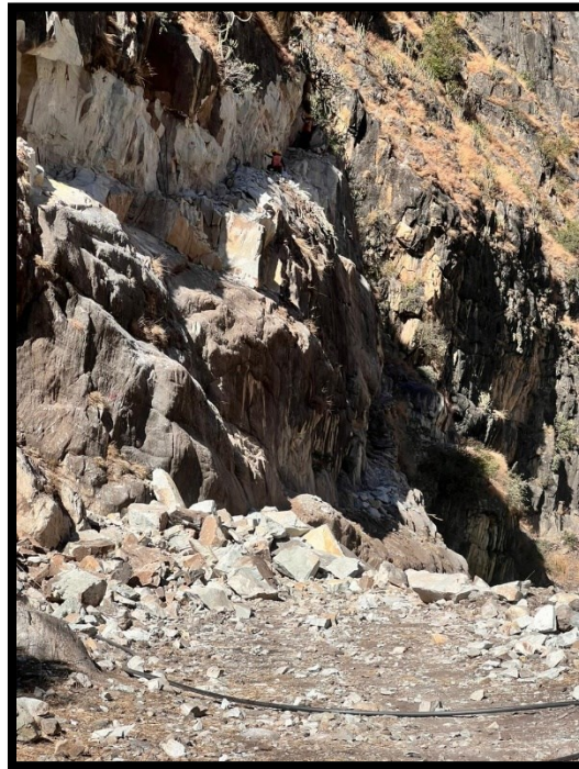
Figure 26: Blasting of Rock along the access Road
