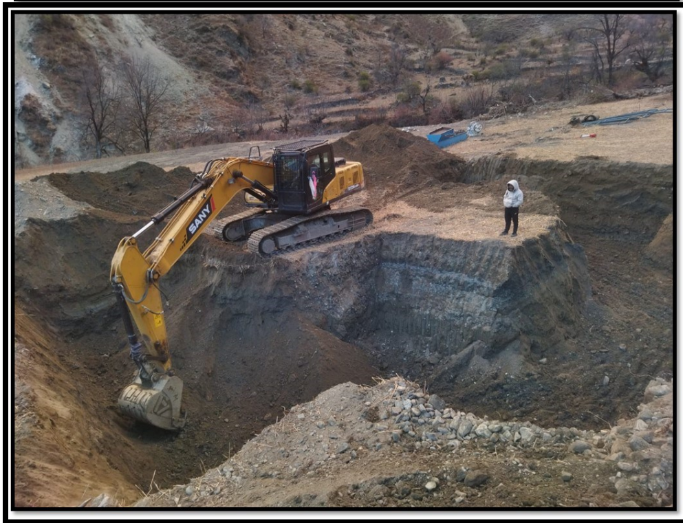
Figure13: Layout and Excavation on Foundation of Camp Facility at head works
