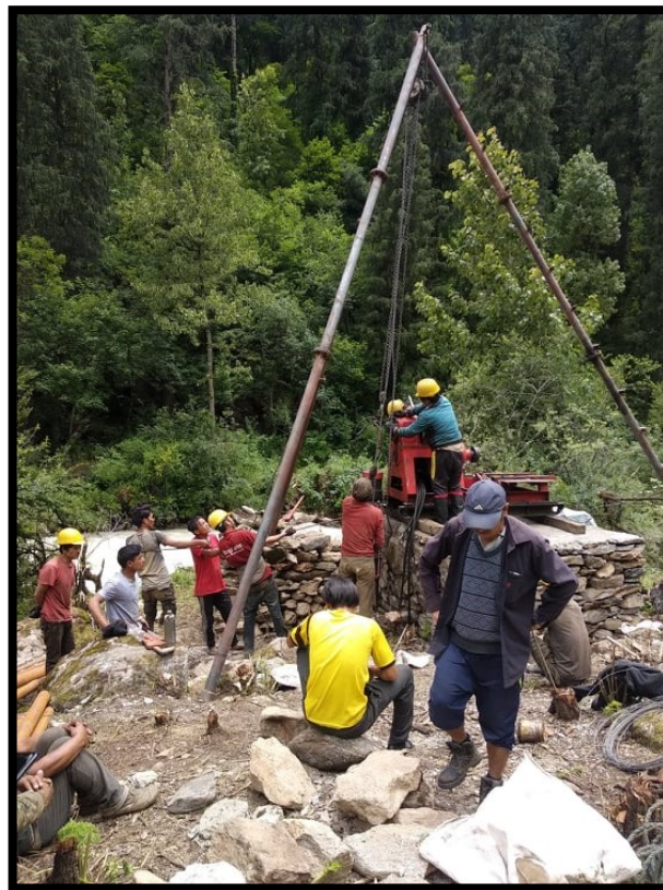
Figure 2: Drilling For Geotechnical Study
