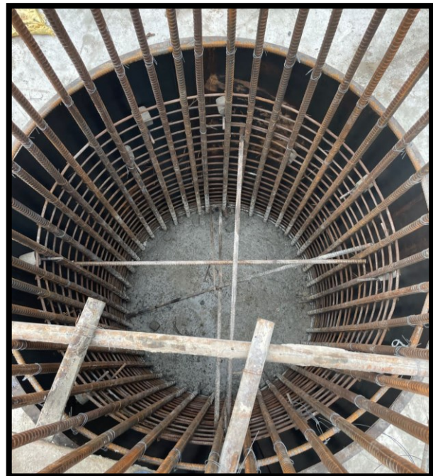
Figure 30:: Construction of Right Abutment
