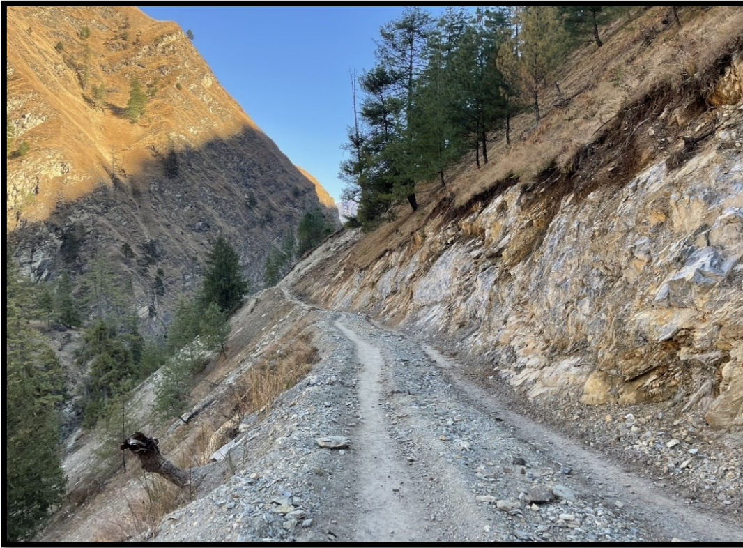
Figure 45: Access Road to the Project Site constructed by IDO, Dolpa
