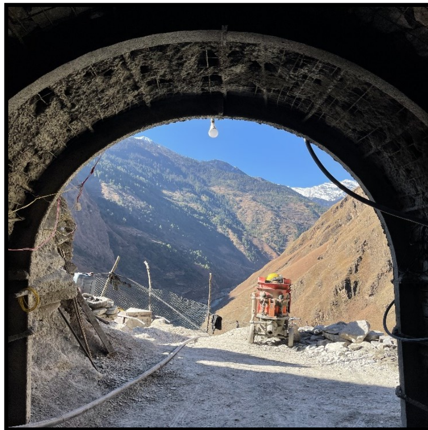
Figure 9: Test Tunnel Photos
