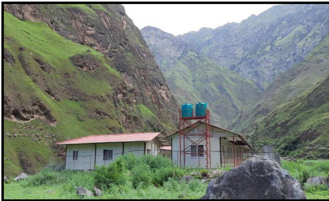
Figure 9: Completed Prefab Office cum Residential Building
