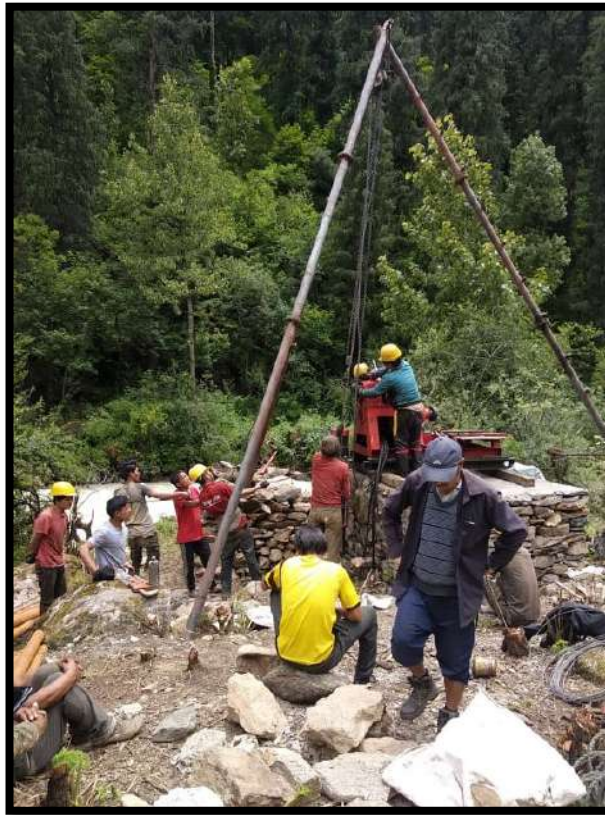
Figure 1: Drilling For Geotechnical Study
