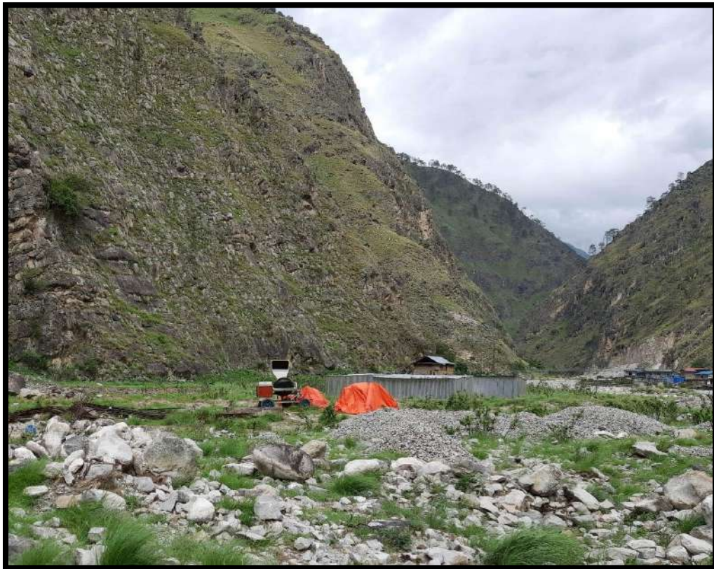
Figure 13: Construction preparation of RCC Bridge and Construction Materials.
