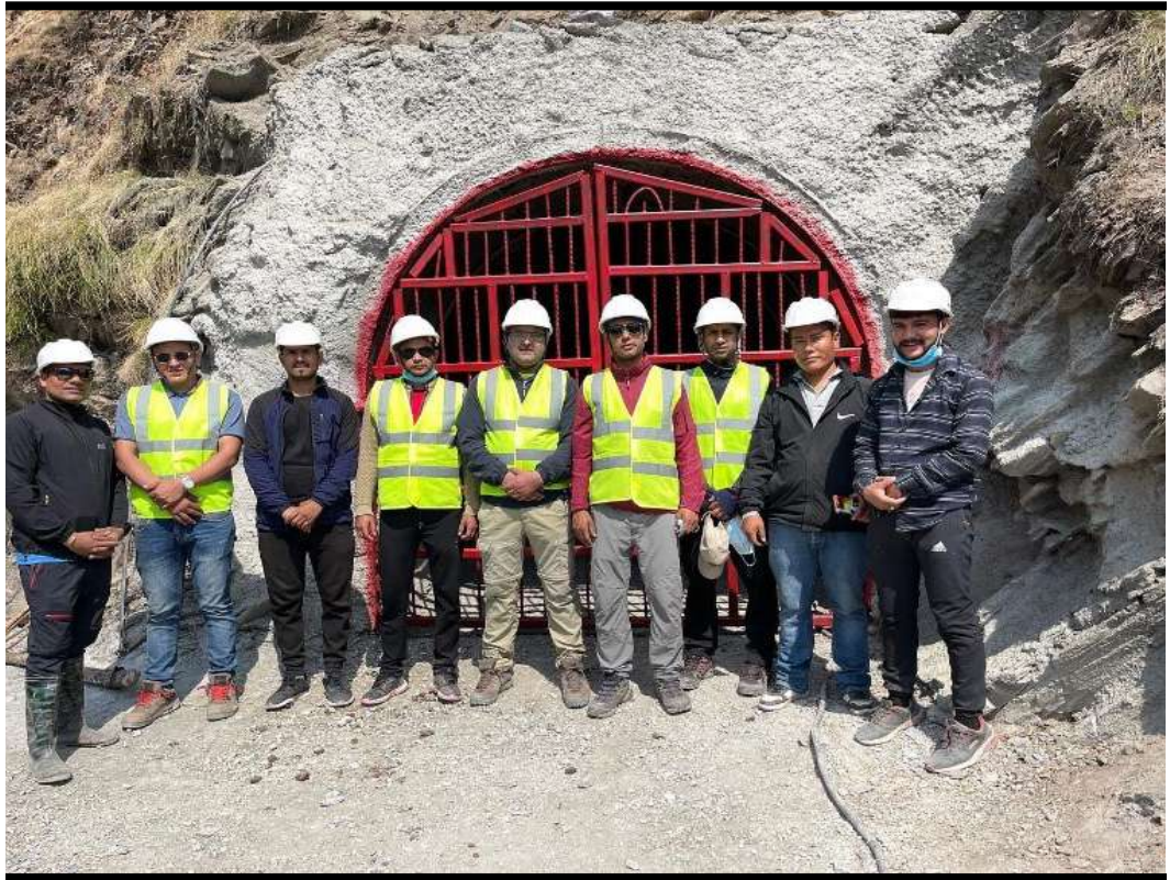
Figure 7: Test Adit Tunnel Completed
