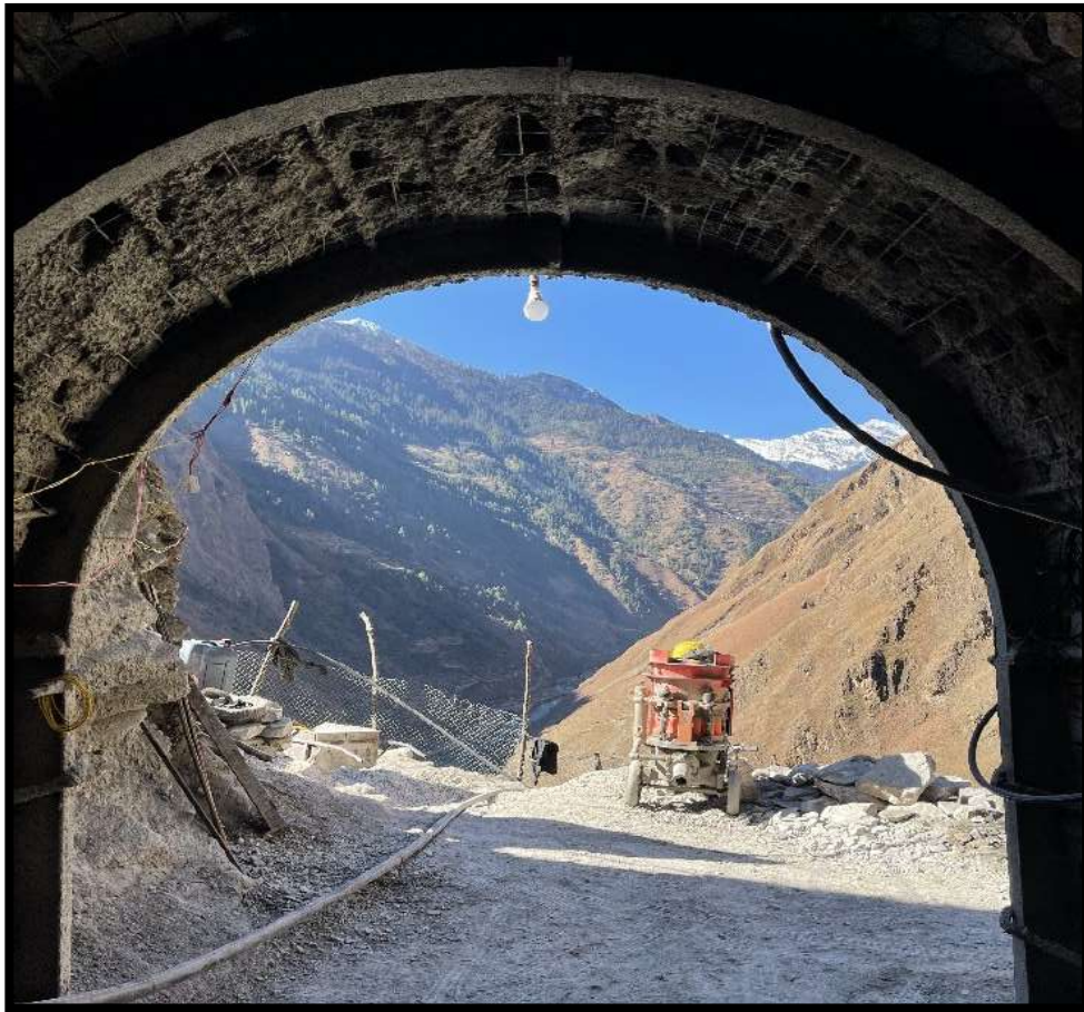
Figure 8: Test Adit Tunnel Photos
