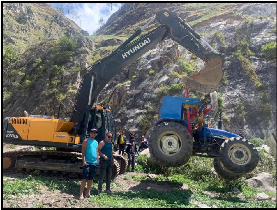
Figure 11 : Carrying and River Crossing of the Equipment of RCC Bridge.
