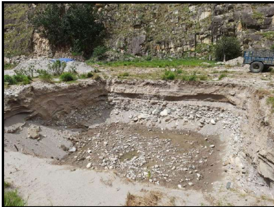
Figure 12: River Training work and Excavation work of RCC Bridge.
