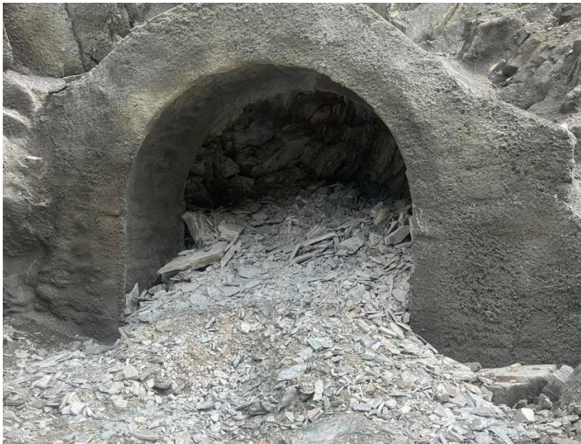
Figure 3: Test Adit Tunnel Under Progress
