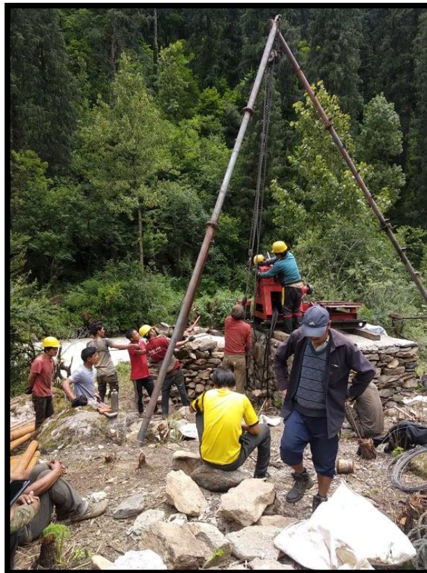
Figure 1: Drilling For Geotechnical Study
