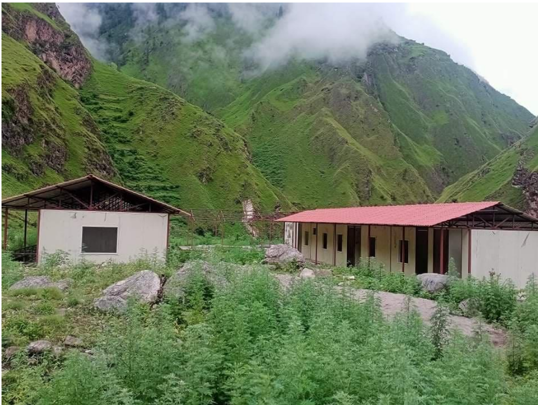
Figure 4: Prefab Office cum Residential Building at final stage of completion.
