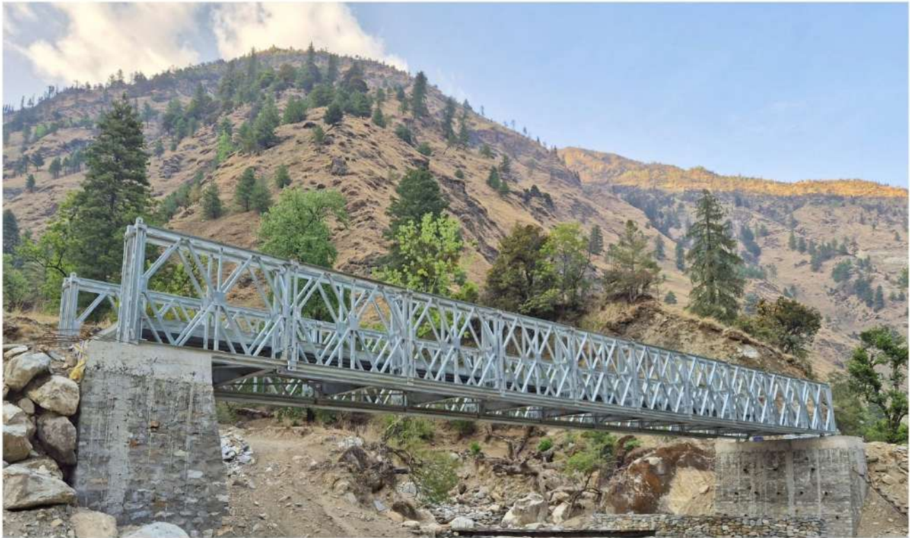
Bailey Bridge 3, Bajhgad
