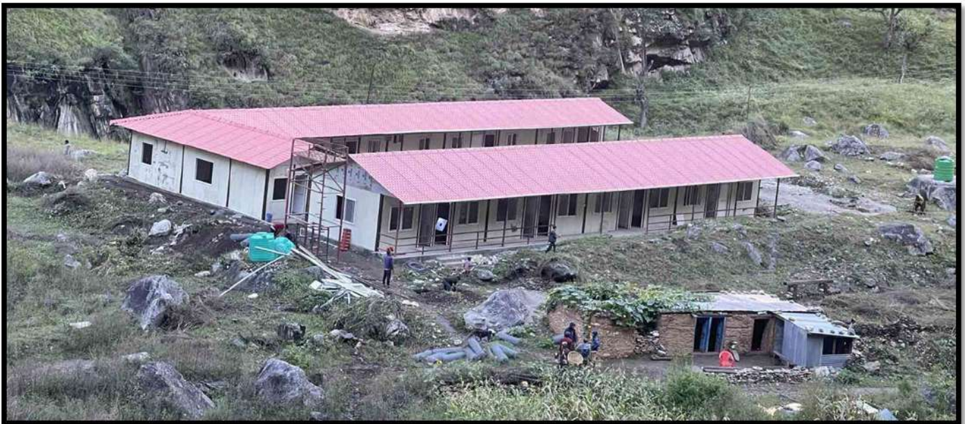
Completed Prefab Office cum Residential Building
