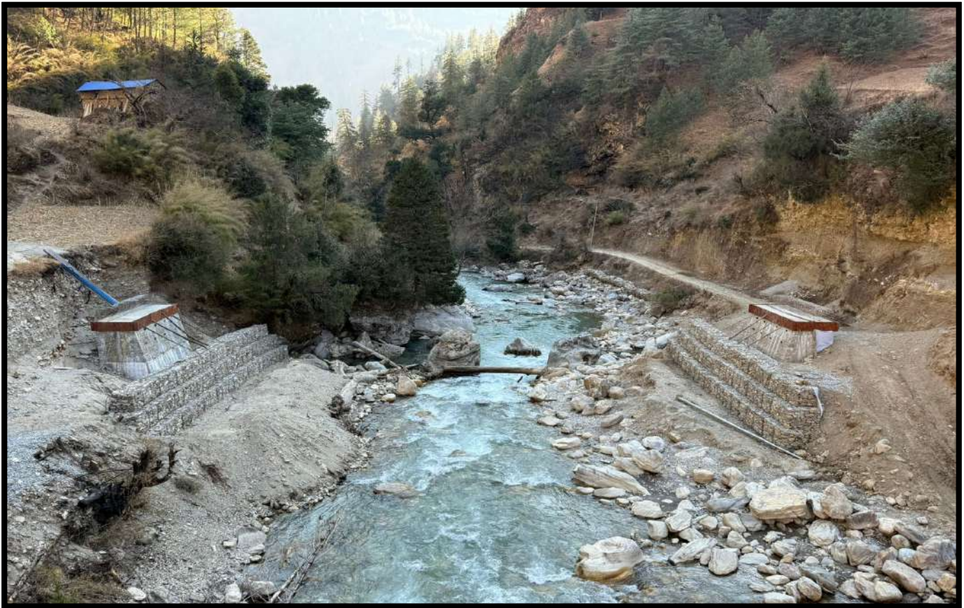
Bailey Bridge 5, Octa Gadpar
